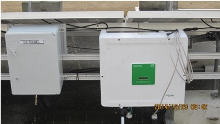
Figure 4. (top) Darfon G320 micro inverters (b) Schneider Conext RL 5000
