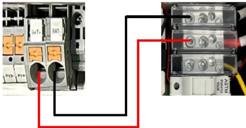
Figure 5.41 Battery Pack to Inverter Power Cable Connection
