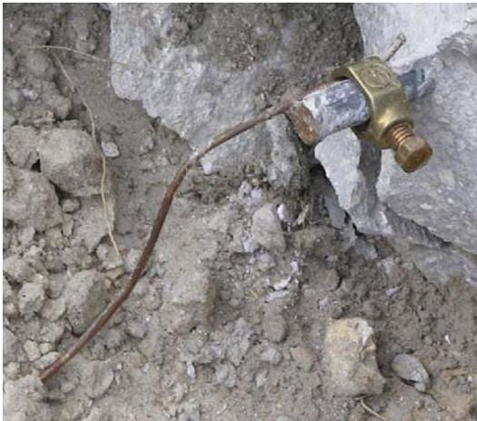
**Figure 5.12** A bonding jumper attached to rebar which is encased in concrete.
