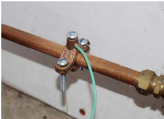
**Figure 5.2** Copper water pipe can serve as an effective ground-fault current path.
