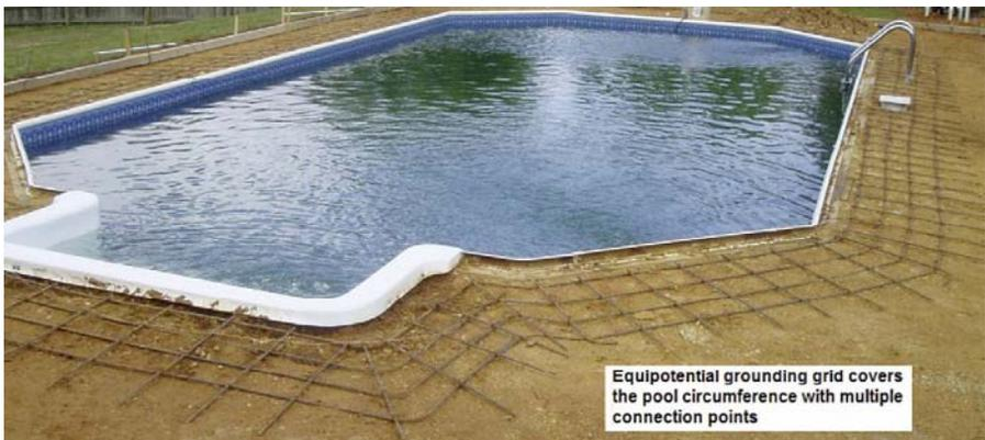
**Figure 6.8** An equipotential grounding grid protects anyone getting out of the pool from shock hazards because they would have the same electrical charge as the pad.
