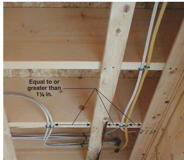
Exhibit 300.3 Nonmetallic sheathed cables adjacent to furring strips in a wood frame structure.
