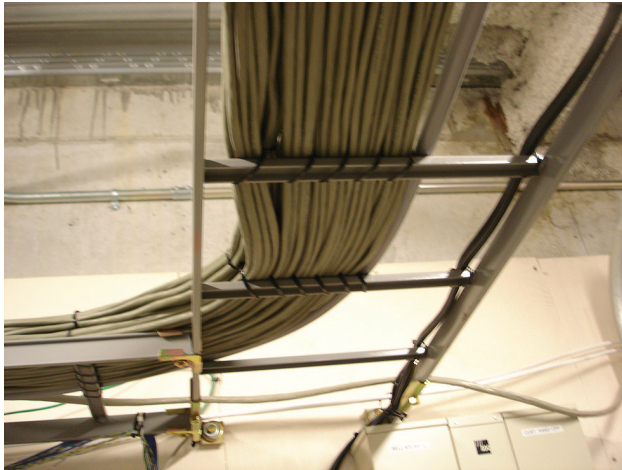
Exhibit 800.7 Overhead ladder-type cable tray containing communications cables.
