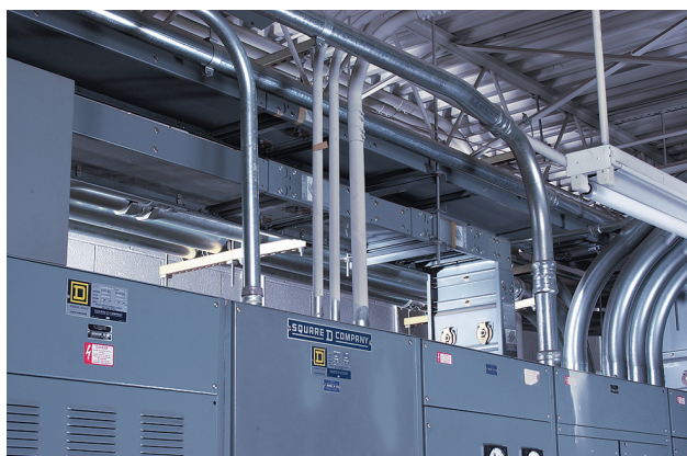
Exhibit 368.1 A 10-ft section of feeder busway.
