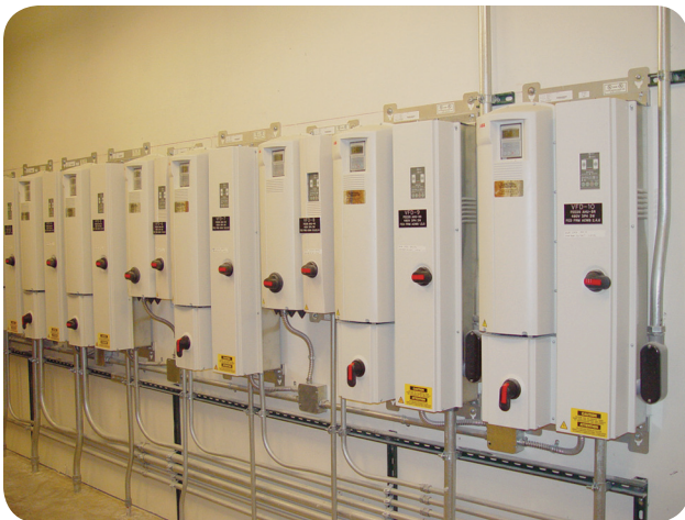
EXHIBIT 430.24 Adjustable-speed drives for air-handling units. These drives provide significant power savings for fan applications. (Courtesy of International Association of Electrical Inspectors)
