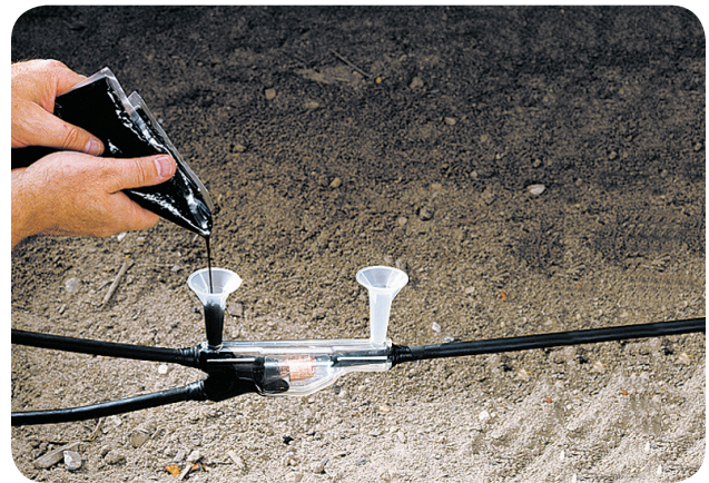
EXHIBIT 300.8 One underground splicing method in accordance with 300.5(E) as well as 110.14(C). (Courtesy of 3M Co., Electrical Markets Division)
