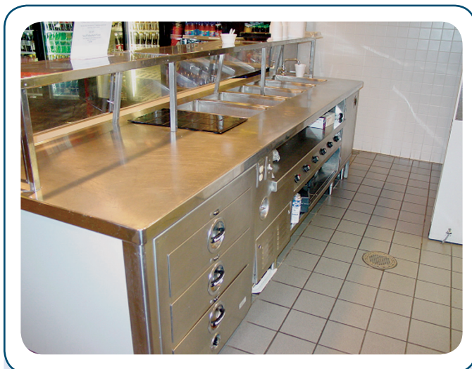
EXHIBIT 220.7 Electrically powered cooking/heating appliance with thermostatic control in a commercial kitchen. Electric appliance loads on feeder and service conductors supplying commercial and institutional kitchens are permitted to be calculated using the demand factors specified in Table 220.56. (Courtesy of the International Association of Electrical Inspectors)
