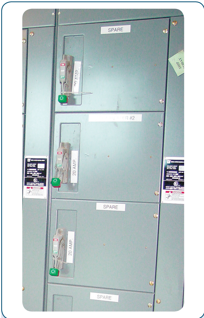
EXHIBIT 90.3 A switchboard with spare circuit breakers installed to facilitate future growth. (Courtesy of the International Association of Electrical Inspectors)
