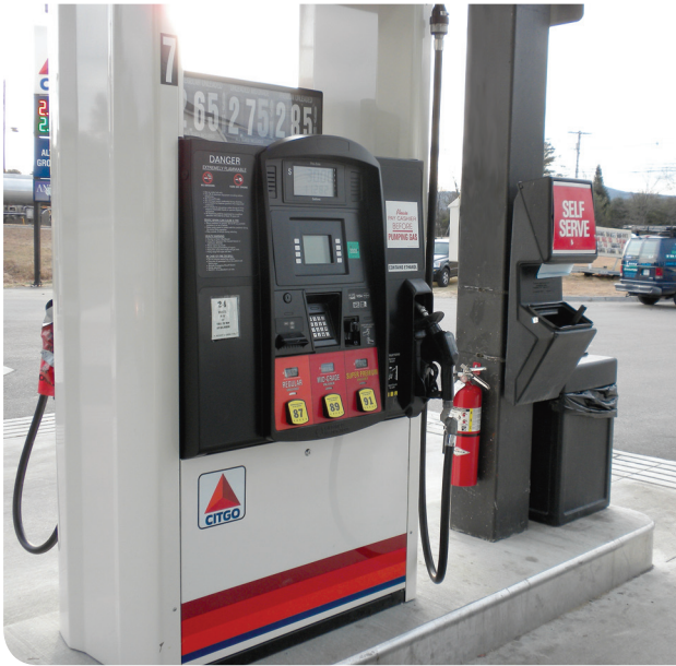
EXHIBIT 514.6 A self-service dispensing island (left) and associated emergency disconnecting means (right).
