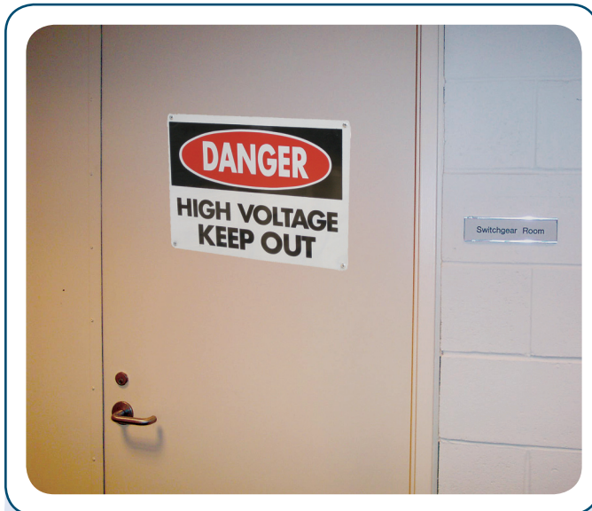
EXHIBIT 100.3 Warning on locked electrical equipment door.
