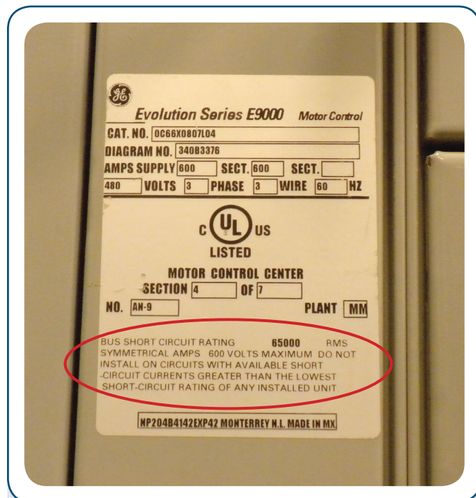
EXHIBIT 100.20 Short-circuit current rating on equipment nameplate.
