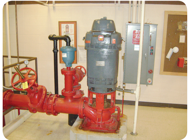
EXHIBIT 695.1 An electric motor specifically listed for fire pump service. (Courtesy of Liberty Mutual Risk Engineering)
