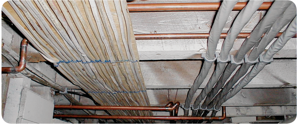
EXHIBIT 334.1 Nonmetallic-sheathed cables and Type SE cables installed in an unfinished basement or crawl space in accordance with 334.15(C).
