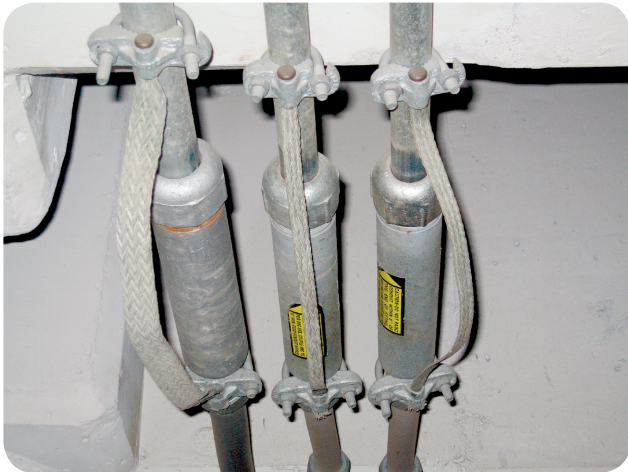
EXHIBIT 100.5 Equipment bonding jumpers installed to maintain electrical continuity around conduit expansion fittings. (Courtesy of the International Association of Electrical Inspectors)
