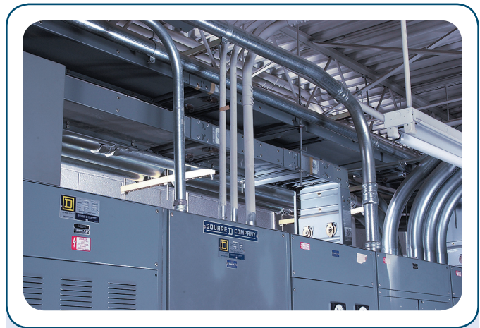
EXHIBIT 368.1 A 10-ft section of feeder busway, which is one type of busway covered by Article 368.
