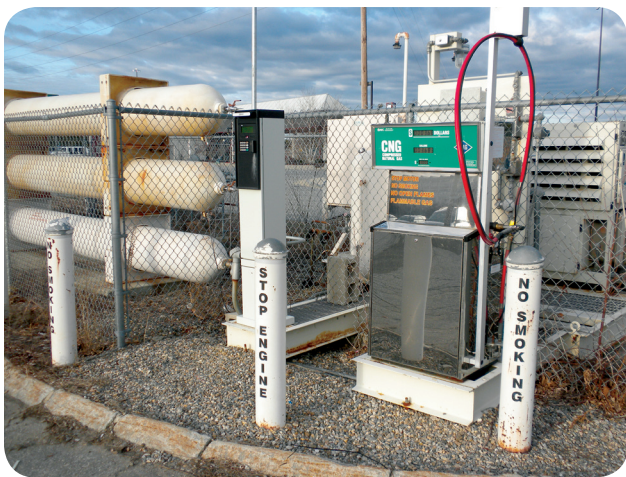
EXHIBIT 500.1 A CNG filling station, which is a Class I location.
