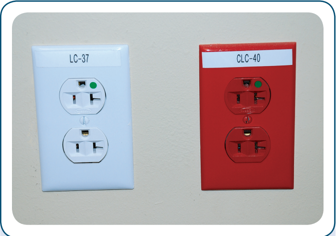
EXHIBIT 517.4 A receptacle from the normal system (left) and the emergency system (right). Note the label that indicates the panelboard and the circuit number. (Courtesy of the International Association of Electrical Inspectors)
