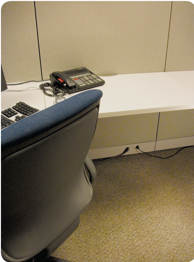
EXHIBIT 605.1 Example of a fixed-type office partition where the supply branch circuit(s) can be connected to the partition wiring either through the top or bottom of the partition.
