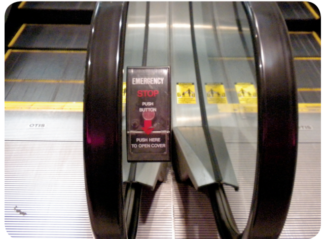
EXHIBIT 620.7 Emergency stop button installed at the escalator location to provide a local means to shut down the equipment in the event of a passenger accident. This is not considered to be the disconnecting means required by 620.51(C)(3).
