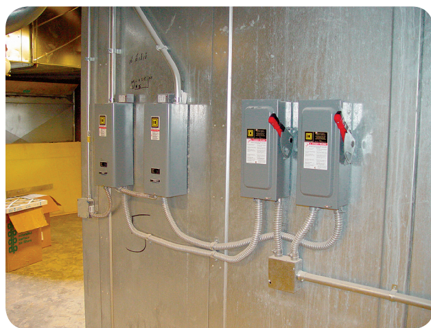
EXHIBIT 430.16 The disconnecting means for each controller, which must be within sight of the controller location per 430.102(A). (Courtesy of International Association of Electrical Inspectors)
