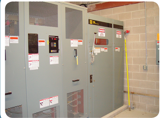
EXHIBIT 110.27 Enclosures of equipment operations at over 600 volts required to have the warning label specified in 110.31(B)(1). (Courtesy of the International Association of Electrical Inspectors)
