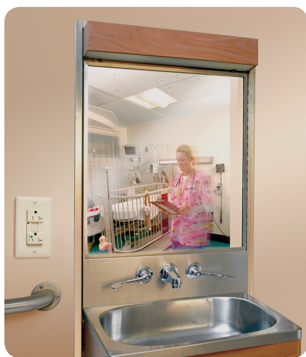
EXHIBIT 517.3 Hospital grade tamper-resistant GFCI in a hospital environment. (Courtesy of Legrand/Pass & Seymour®)
