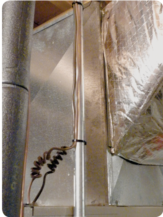
EXHIBIT 300.12 Raceway used to support Class 2 thermostat cables specifically permitted by 300.11(B)(2).
