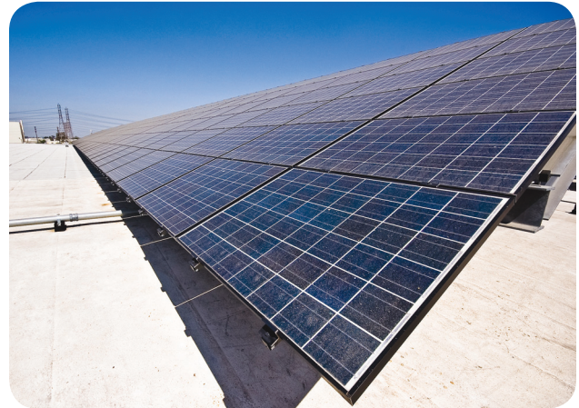
EXHIBIT 690.2 An array composed of multiple modules or panels installed on a support structure and foundation. (Courtesy of NECA)
