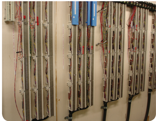
EXHIBIT 800.3 Two examples of punch blocks used on a private automatic branch exchange.
