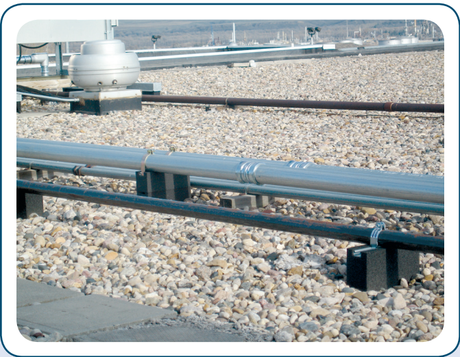
EXHIBIT 310.4 An IMC conduit crossing a rooftop and exposed to sunlight. (Courtesy of the International Association of Electrical Inspectors)
