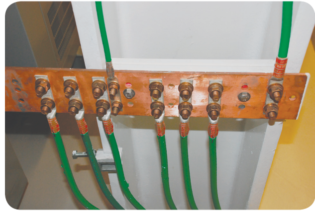
EXHIBIT 250.15 Listed connectors used to connect the common grounding electrode conductor and individual taps to a centrally located copper busbar with a minimum dimension of ¼ in. thick by 2 in. wide.
