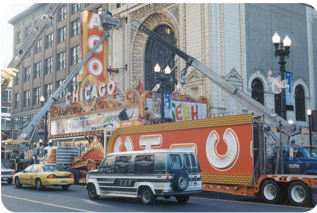
EXHIBIT 600.1 Example of a section sign where the subassemblies are joined together to form a single sign. (Courtesy of Kieffer & Co. Inc.)
