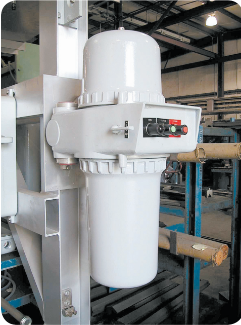
EXHIBIT 501.15 An explosionproof enclosure for a motor control starter and circuit breaker. (Courtesy of Appleton Electric Co., EGS Electrical Group)
