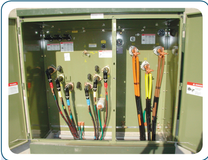
EXHIBIT 490.4 Open view of a tamperproof pad-mount transformer for loop-feed application with load-break elbow connectors. The high-voltage compartment on the left has bayonet fusing and a load-break transformer on/off switch, which are both hot-stick operated. (Courtesy of Schneider Electric)
