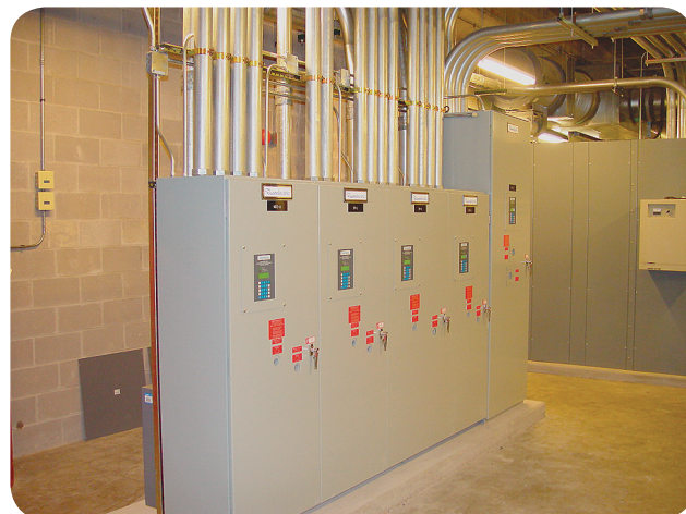
EXHIBIT 110.15 Equipment location that is free of storage to allow the equipment to be worked on safely. (Courtesy of the International Association of Electrical Inspectors)
