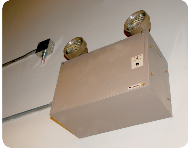
EXHIBIT 700.9 Self-contained, fully automatic unit equipment for operating emergency lighting located on the unit or for remotely located exit signs or lighting heads. (Courtesy of the International Association of Electrical Inspectors)
