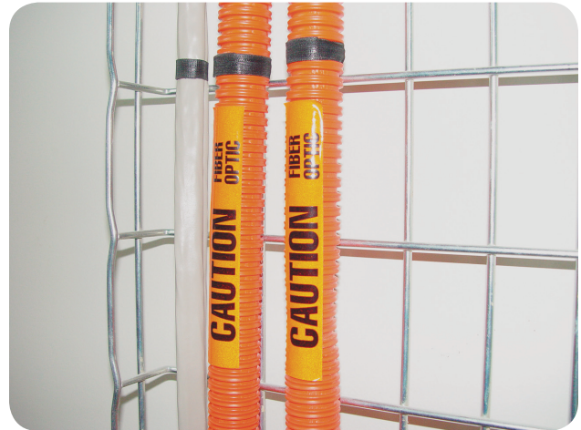
EXHIBIT 770.3 Typical optical fiber raceways. (Courtesy of the International Association of Electrical Inspectors)
