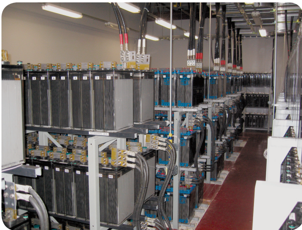
EXHIBIT 480.1 A well-arranged battery room with batteries installed on corrosion-resistant racks. (Courtesy of the International Association of Electrical Inspectors)
