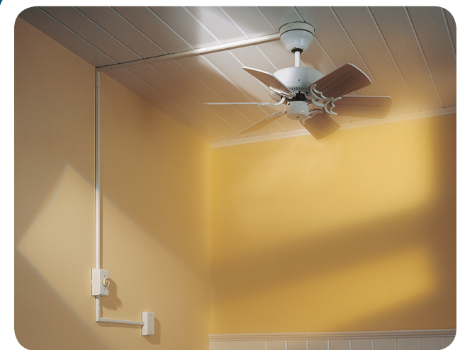
EXHIBIT 386.2 Use of surface metal raceway and associated fitting to supply ceiling-paddle fan and associated speed control.
