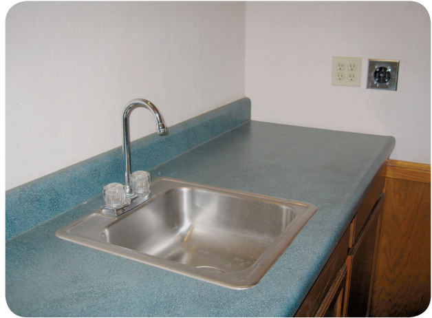
EXHIBIT 210.16 GFCI protection required for single-phase, 125 volt, 15 ampere rated duplex receptacles installed within 6 ft of a sink.
