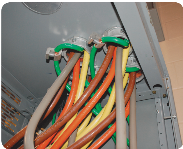
EXHIBIT 215.2 Different colors being used to identify each ungrounded line or phase conductor of a nominal voltage system.
