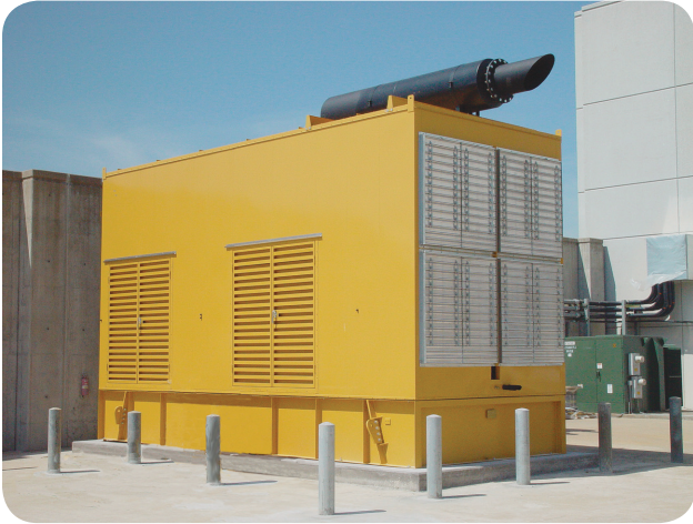
EXHIBIT 700.8 Alternate source of power in a heated and secure enclosure that is located in an area not subject to flooding. (Courtesy of the International Association of Electrical Inspectors)
