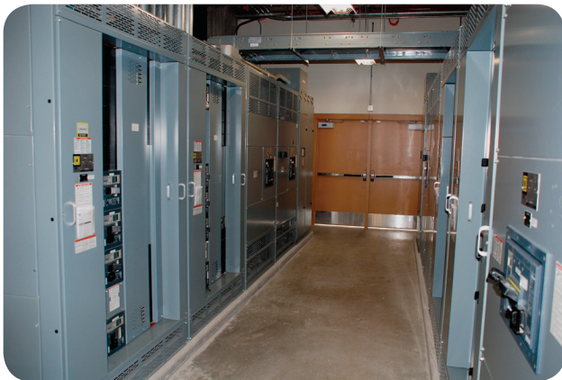
EXHIBIT 110.21 An installation of large equipment showing one of the required exits. (Courtesy of the International Association of Electrical Inspectors)
