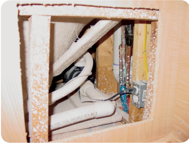
EXHIBIT 680.15 Hydromassage bathtub circulating pump motor and supply receptacle located per 680.73. (Courtesy of the International Association of Electrical Inspectors)
