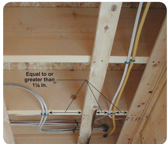
EXHIBIT 300.2 Nonmetallic sheathed cables adjacent to furring strips in a wood frame structure in accordance with 300.4(D).
