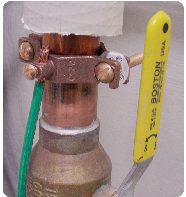
EXHIBIT 250.32 An application of a listed ground clamp.
