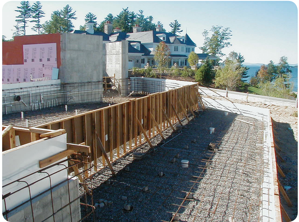
EXHIBIT 680.10 A poured-concrete pool with structural reinforcing steel that serves as the pool shell bonding grid.
