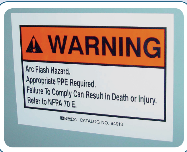
EXHIBIT 110.7 One example of an arc flash warning sign required by 110.16. (Courtesy of the International Association of Electrical Inspectors)
