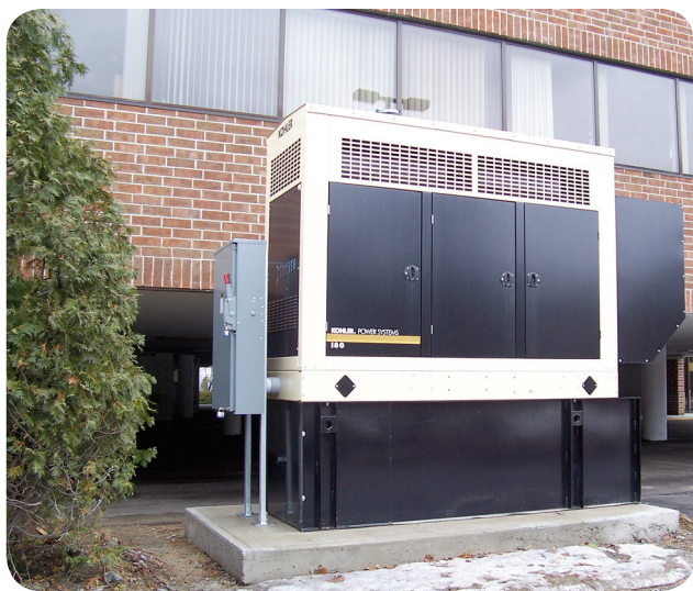
EXHIBIT 225.6 Disconnecting means for alternate source feeder supplying emergency, legally required standby, or optional standby loads or a combination of the three.
