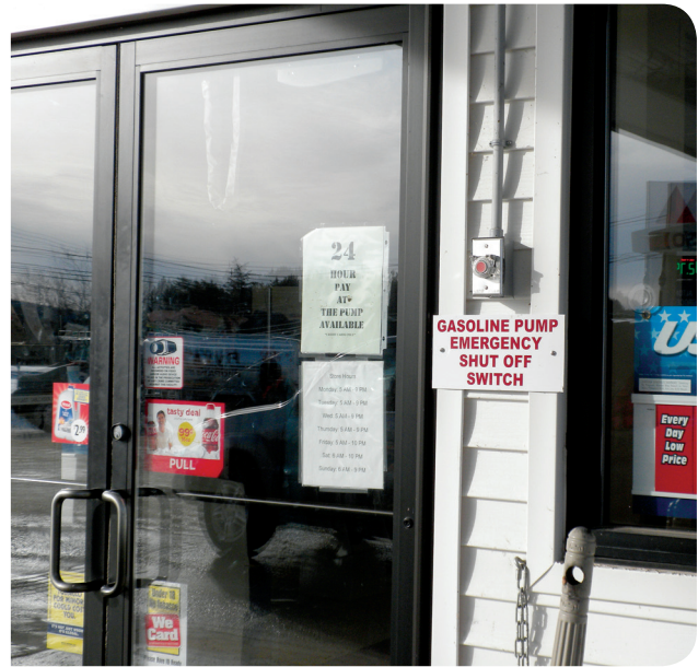
EXHIBIT 514.6 A self-service dispensing island (left) and associated emergency disconnecting means (right).
