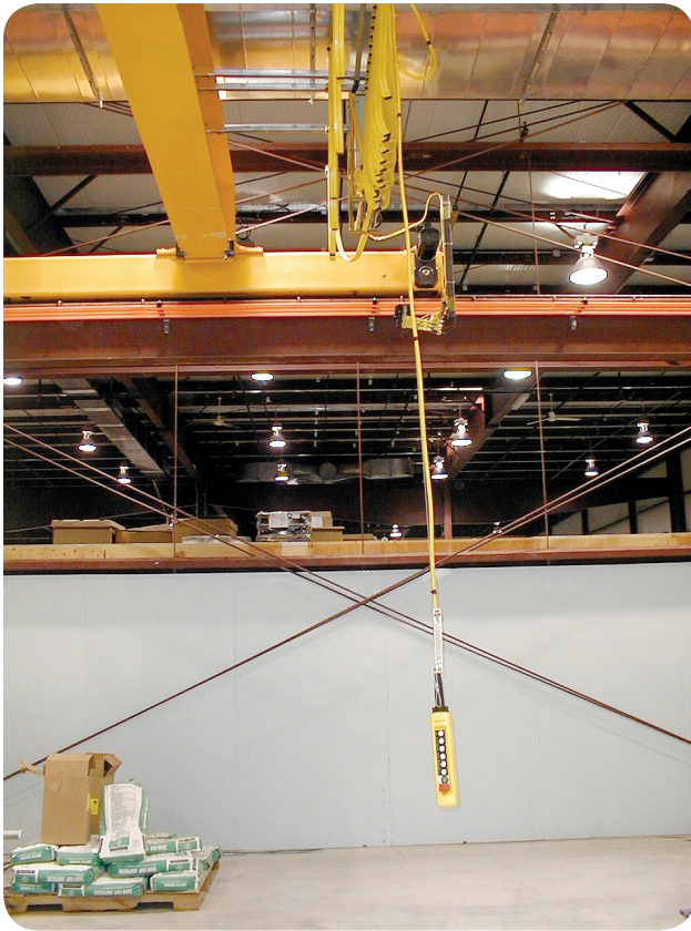
EXHIBIT 610.2 A suitable strain relief grip for a cord-suspended pushbutton station.
