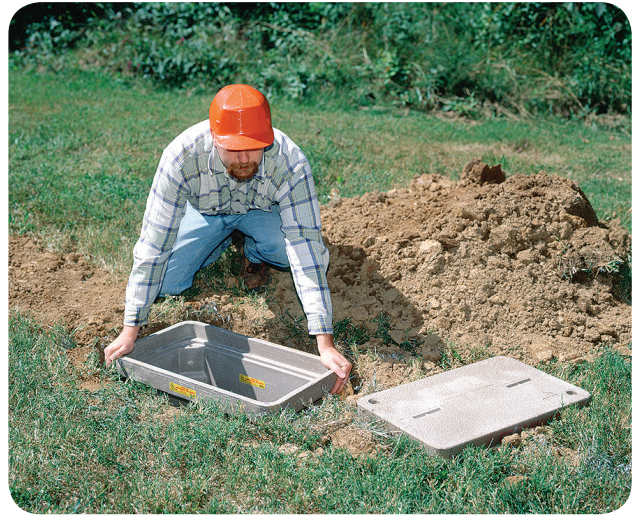
EXHIBIT 100.12 Example of handhole enclosure installation. (Courtesy of Quazite®/Hubbell Lenoir City, Inc.)
