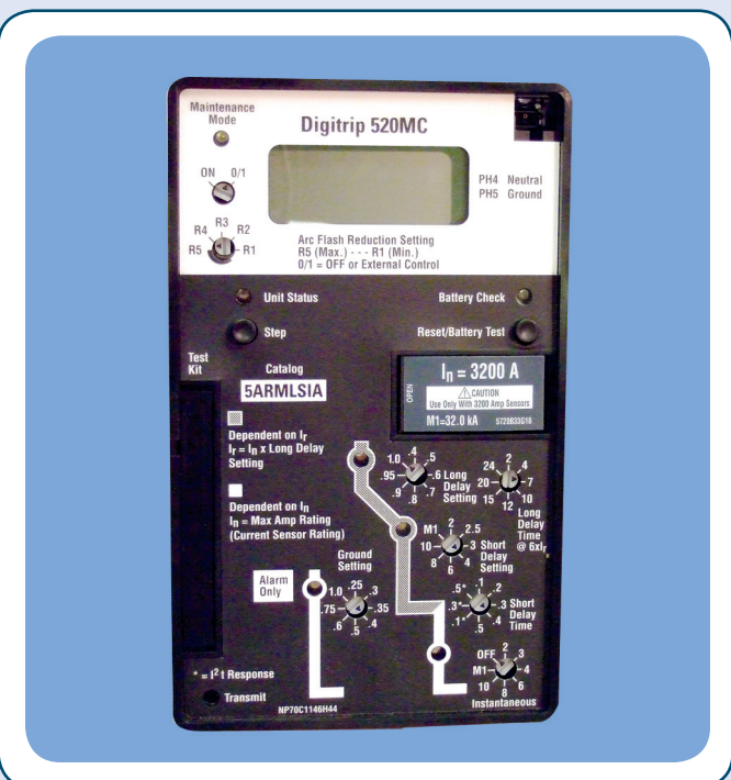
EXHIBIT 240.15 An electronic trip unit for a circuit breaker that has its instantaneous setting set to “Off” and that incorporates an energy-reducing maintenance setting. (Courtesy of Eaton Corporation)
