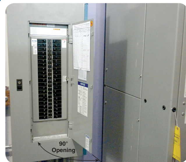
EXHIBIT 110.14 Illustration of requirement that the depth of working space must be sufficient to allow a full 90 degree opening of equipment doors in order to ensure a safe working approach.
