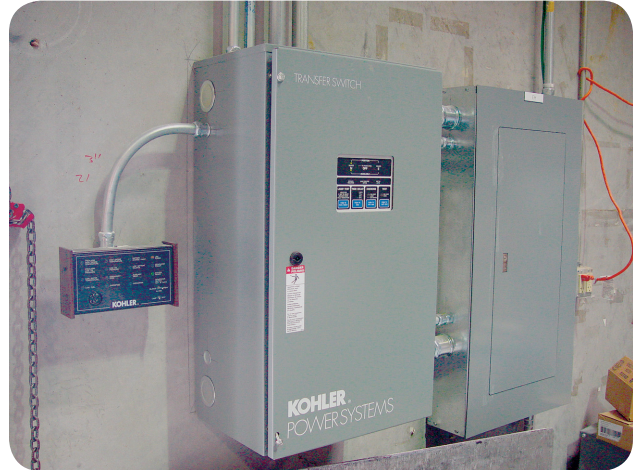
EXHIBIT 700.1 An emergency system transfer switch. (Courtesy of the International Association of Electrical Inspectors)
