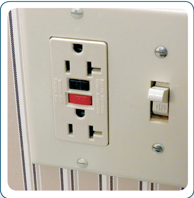
EXHIBIT 210.8 A 15-ampere duplex receptacle with integral GFCI that also protects downstream loads.
