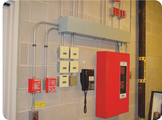
EXHIBIT 760.1 Typical fire alarm control unit. (Courtesy of the International Association of Electrical Inspectors)
