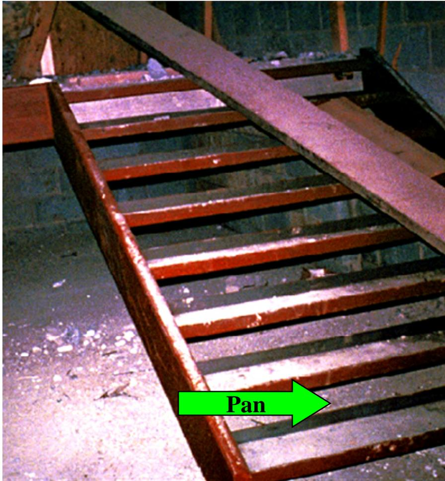
**Only use pan stairs if filled with filler material at least to the top edge of each pan.**
