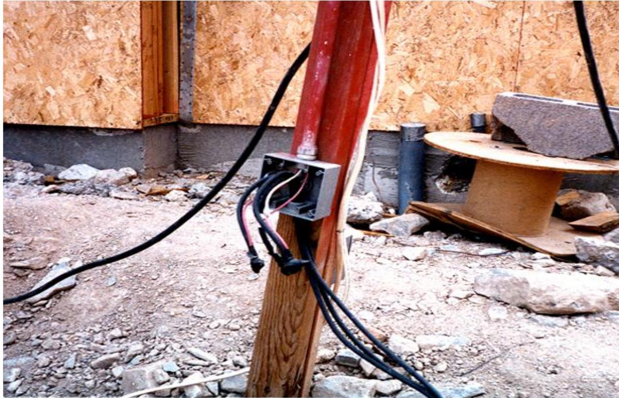
Cover removed from wiring or breaker box
