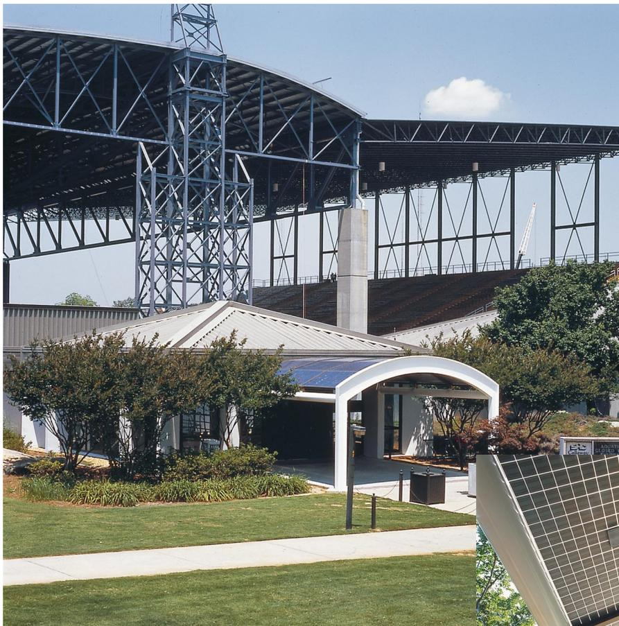
*The entranceway canopy of the Aquatic Center at Georgia Institute of Technology is roofed with a 4.5 kW array of Solarex PowerWall™ MSX-240/AC laminates. With their integrated inverters, these laminates provide grid-synchronized AC power. They use an optional clear Tedlar® backing material which emphasizes the precision of solar cell placement and provides soft natural lighting under the canopy.*
