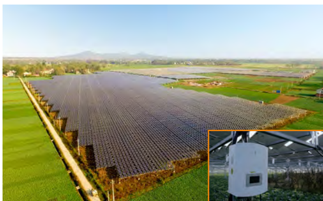
Hubei Guanyin Agricultural-photovoltaic hybrid PV plant 20MW
