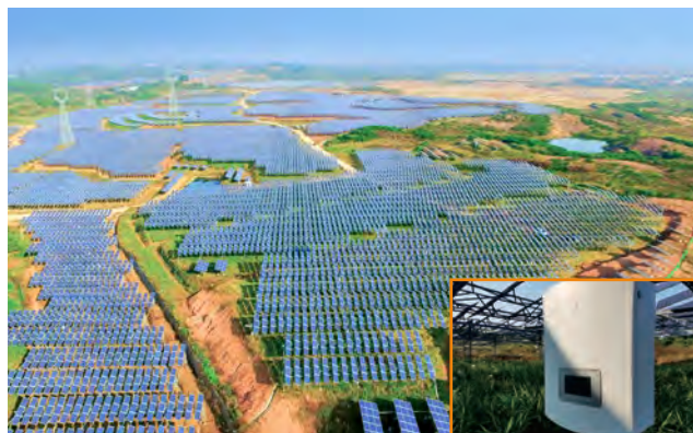
Zhejiang Hangbu Agricultural-photovoltaic hybrid PV plant 30MW
