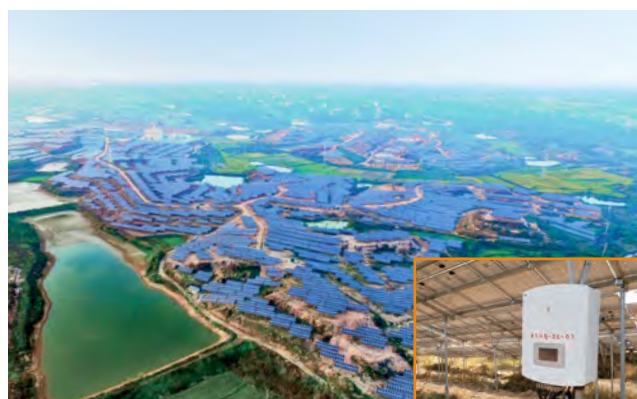
Zhejiang Longyou Agricultural-photovoltaic hybrid PV plant 25MW
