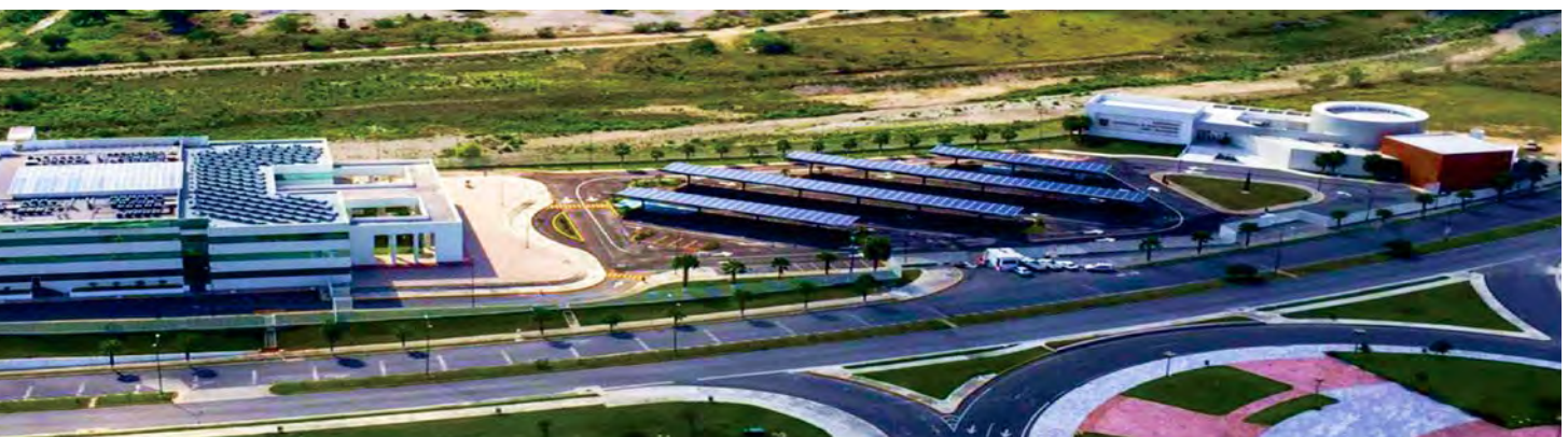
Mexico-Tamaulipas Carport, Mexico 5MW
