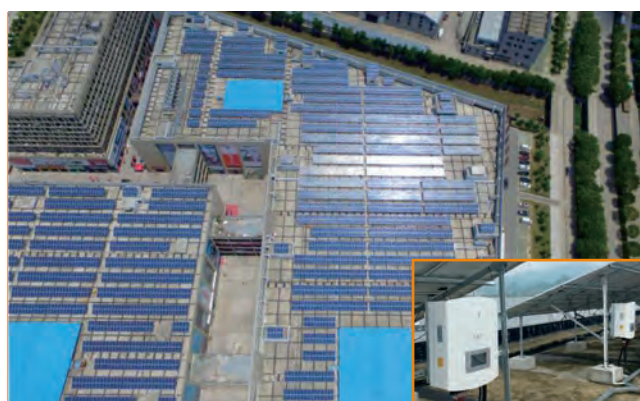
Ninghai AB hall, modern home plaza 1.53MW
