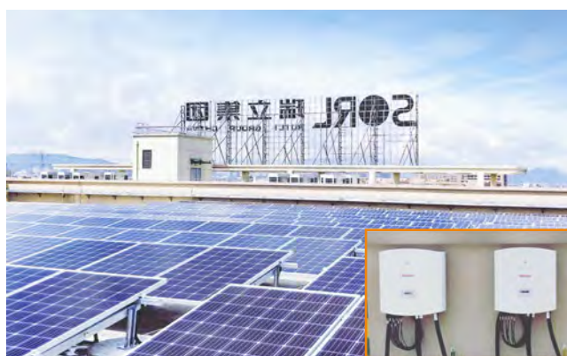
Zhejiang SORJ 3.9MW
