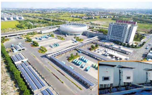
Zhejiang PINGHU Bus Station 472kW
