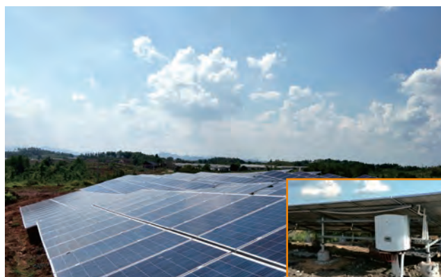
Jiangxi Ganzhou PV Plant 3.5MW
