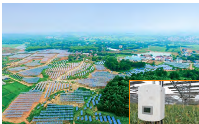
Quzhou Qinghu Agricultural-photovoltaic hybrid PV plant 20MW
