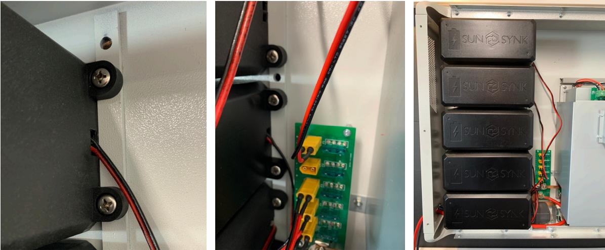
**A minimum battery cable size of 35mm diameter is recommended.**
