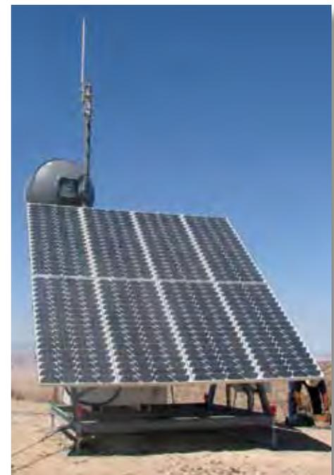
*This 1200 watt SunWize Power Station located in a remote location, powers telemetry equipment*
